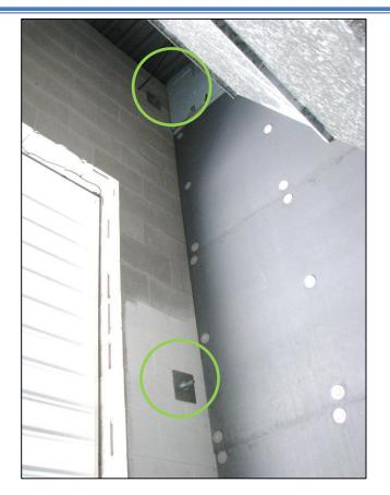
Figure 10: Through bolts in concrete
