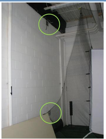
Figure 8: Through-bolts for mounting antenna mast
