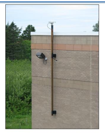
Figure 7: Antenna mast connected to a load bearing wall
