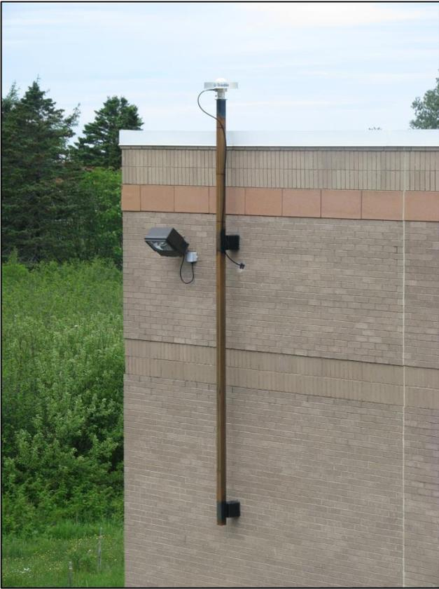
Figure 7: Antenna mast connected to a load bearing wall
