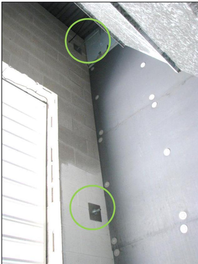
**Figure 10: Through bolts in concrete**
