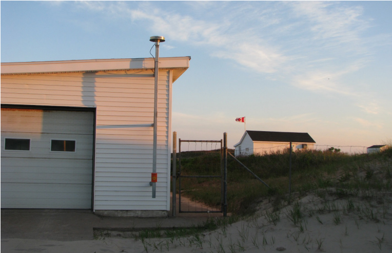
Fig 8 Nova Scotia Active Control Station located on the Garage at Main Station, Sable Island.
