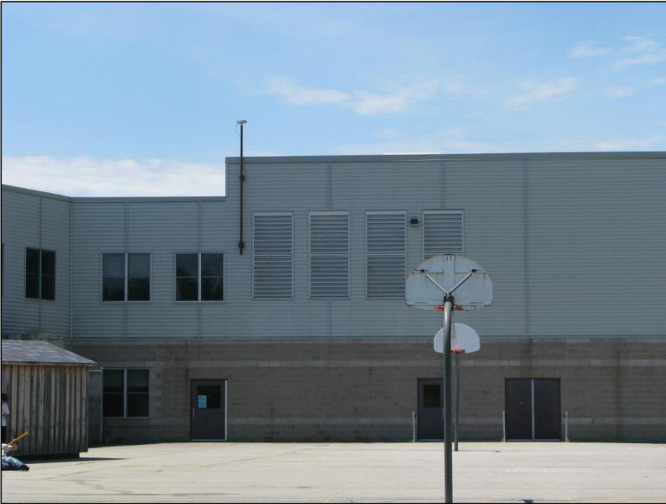
Figure 9: Metal Siding with Concrete Inner Wall Installation
