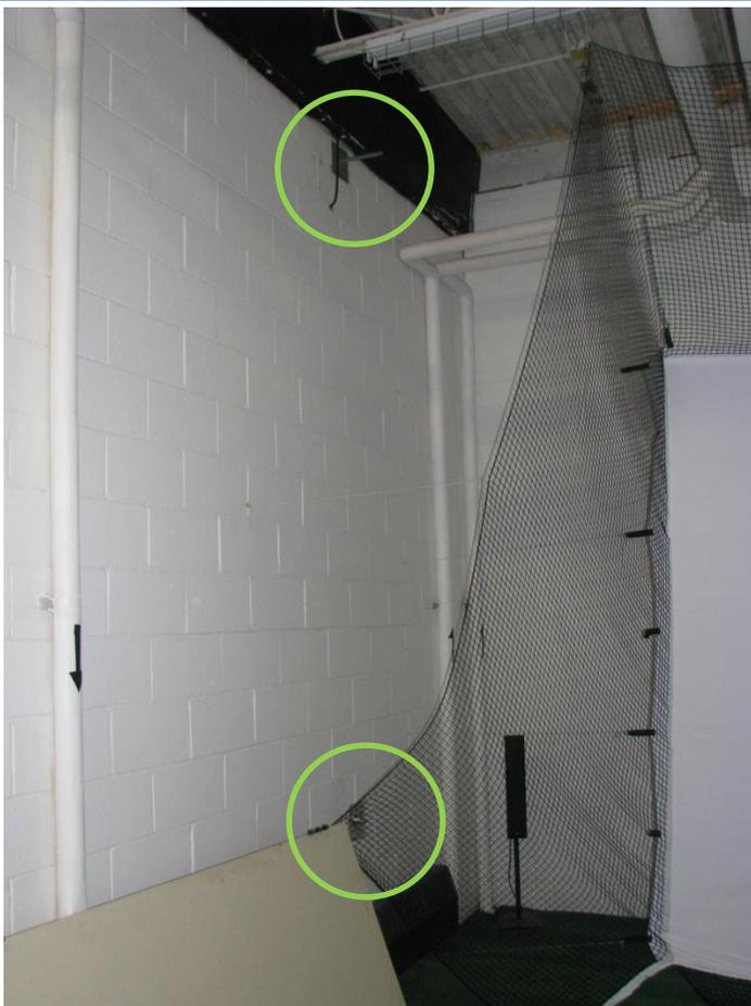
**Figure 8: Through-bolts for mounting antenna mast**
